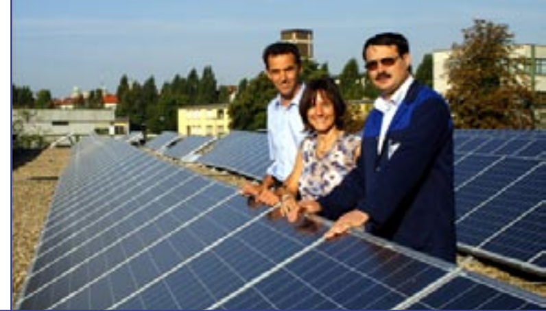
Augsberg, Germany has installed solar panels to supplement their depot requirements for energy.
